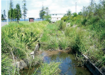
Vegetation planted in a concrete drainage channel to improve water quality
